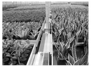
Figure 5: Fiwihex heating and cooling in a all year closed horticulture greenhouse
