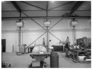
*Figure 6: Fiwihex very low temperature heating and cooling device in a machine factory*
